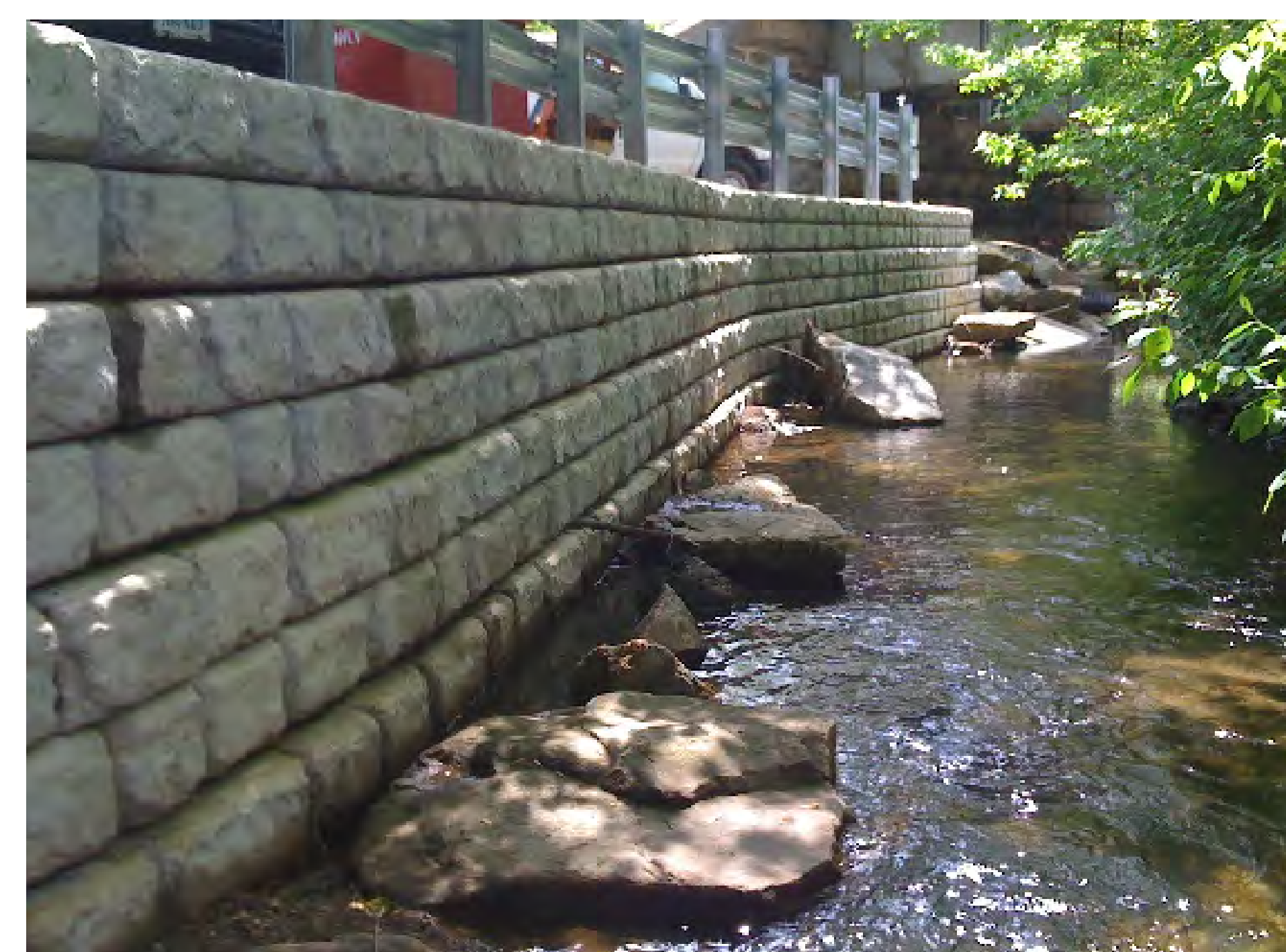
TOE ROCK WALL PROTECTION
